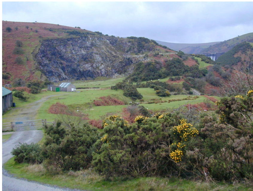
The southern and larger aplite quarry and some of the surviving buildings; with Meldon Dam beyond (Photo: Kevin Page 2005)
